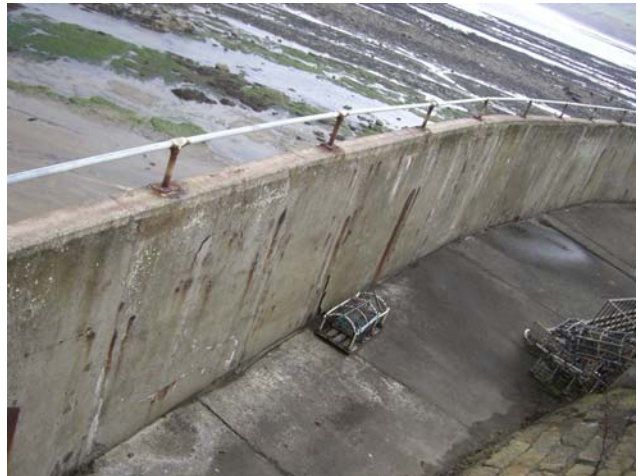
Plates T4: Views at the top of the wall, showing a small parapet, with handrail and paved walkway of extremely variable width.
