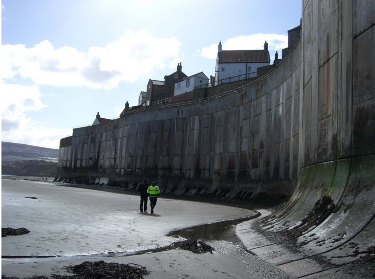
Plate T1: General view of the wall from the northern end.
